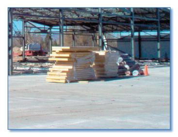
Structurally-insulated panels provide a continuous insulation level that traditional framing can't match.
