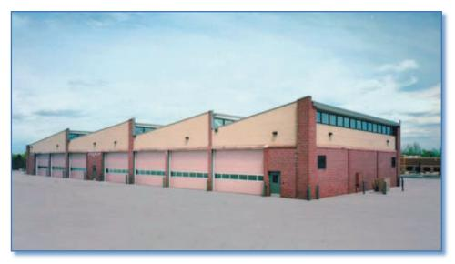
An energy saver with warm floors and daylighting—the new Utilities vehicle storage building is an example of cutting-edge green building techniques.
